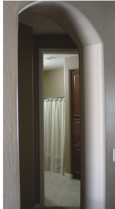
10" ETS with 90° Elbow installed on Side Wall
